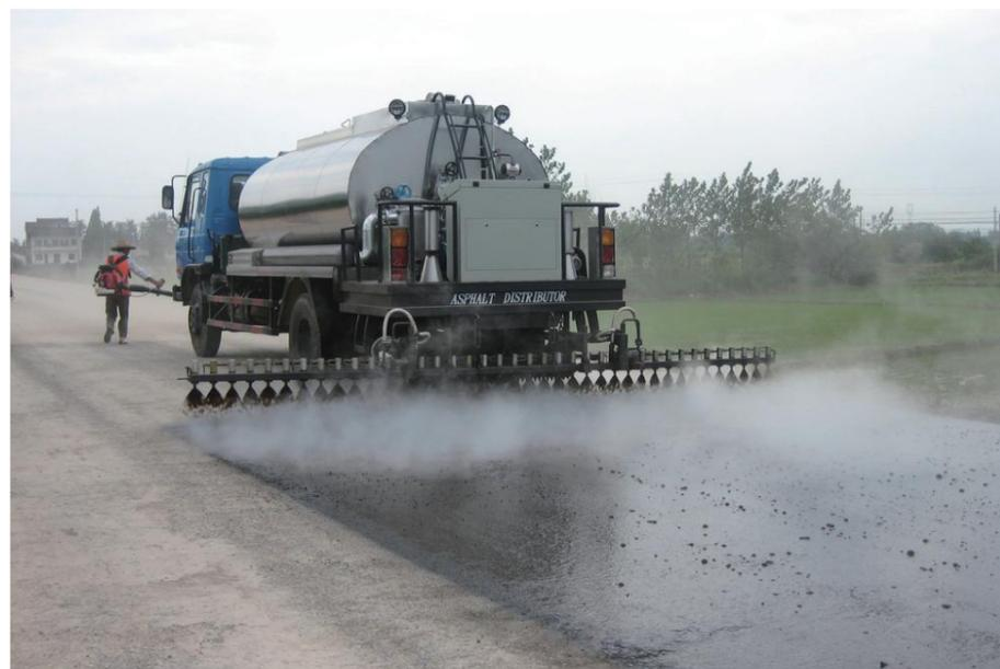
Automatic Bitumen Sprayer in Australia
